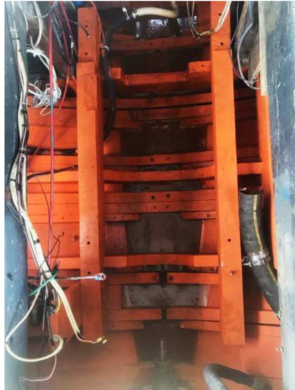
Engine bilge with engine out, floors and frames inspected and re-painted
